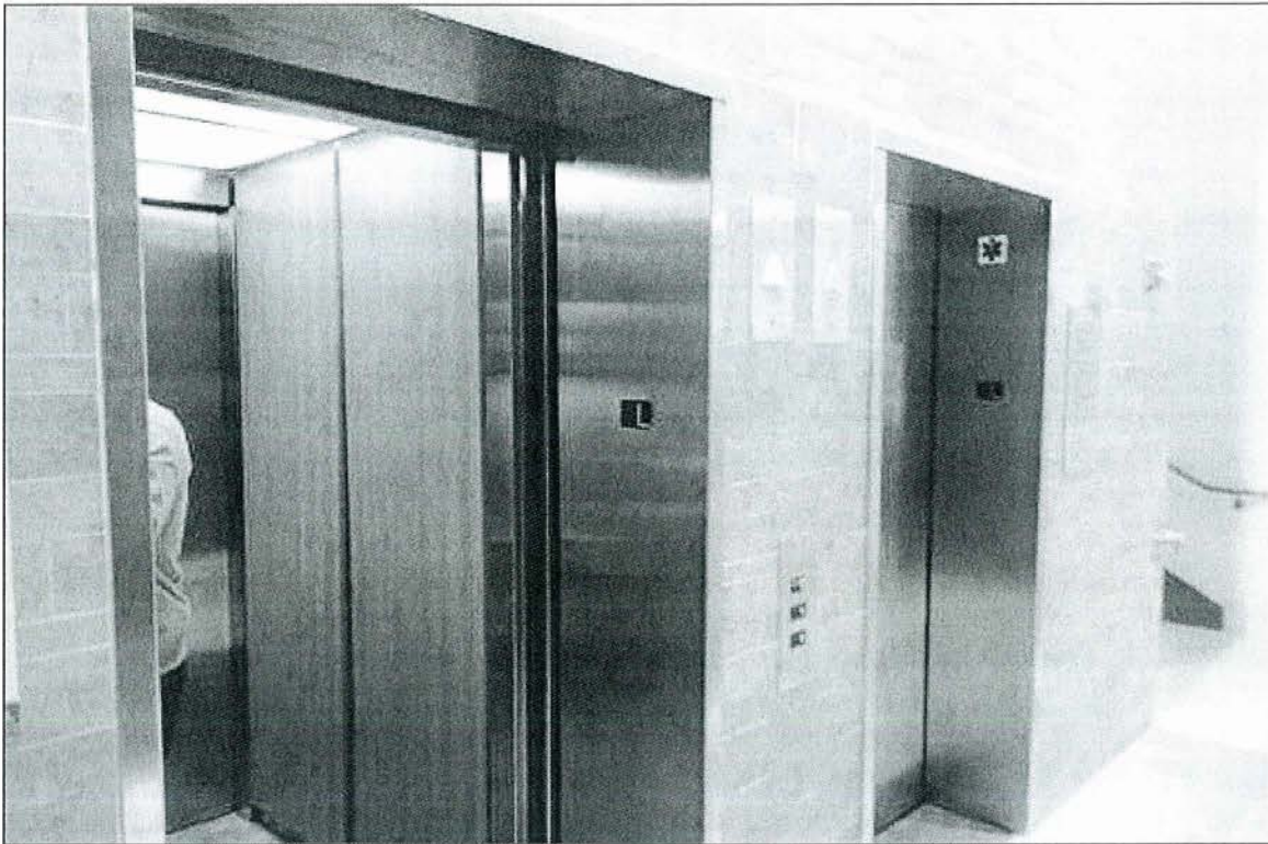
Subject Elevator Bank
