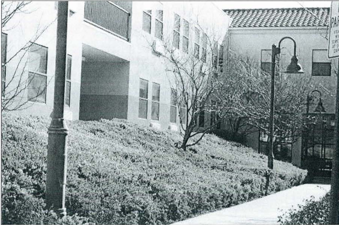
Sidewalk and Landscaped Area around the Southern Side of the Subject
