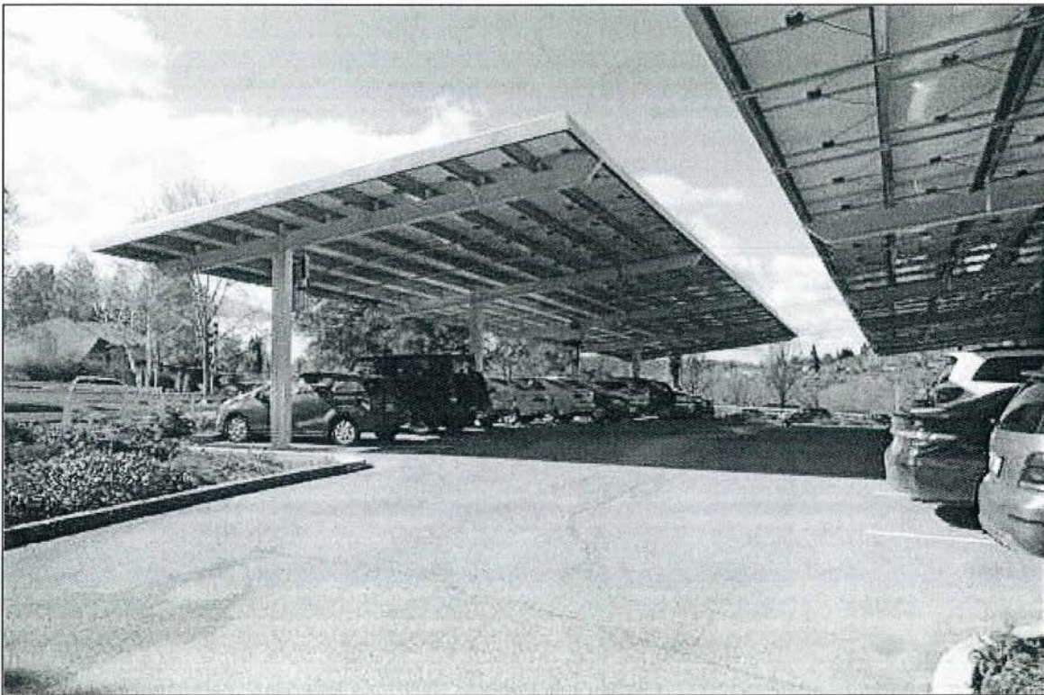
Additional Parking Area at the Southwest Corner of the Site (note solar panels on the rooves)
