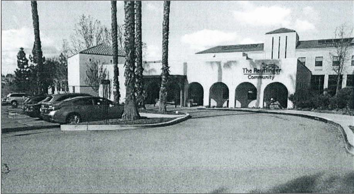
Subject Front Entry Area of Building
