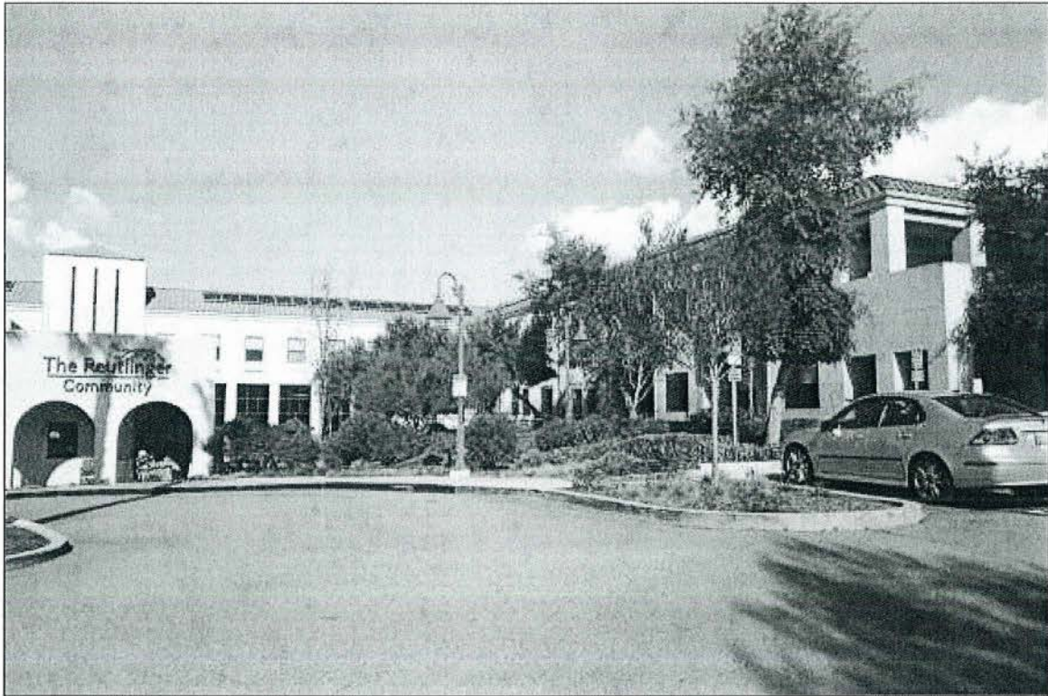
Subject One and Two-Story Building Areas from Entry Driveway
